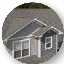
Roofing and Ventilation
